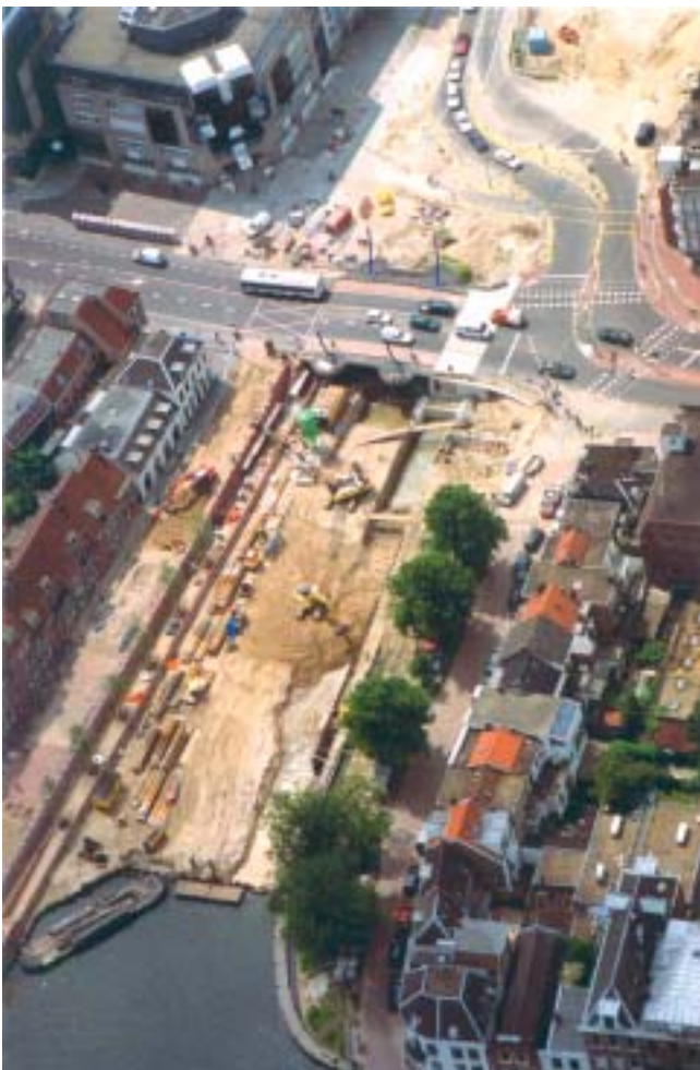
Reinstatement of the Encircling Canal, Utrecht.
